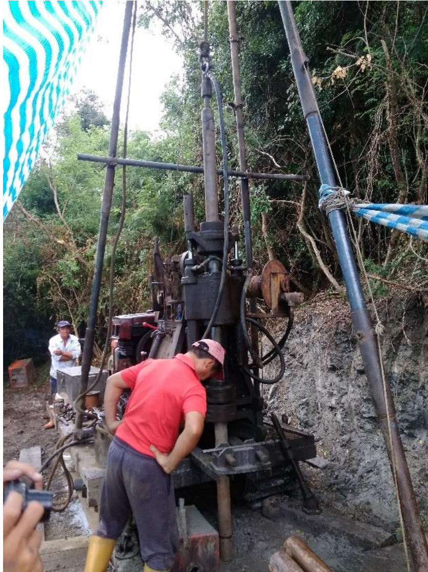
Figure 2.3 Photograph of the operation of the drilling machine.
